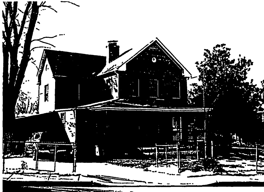
Figure 17. The William and Martha Smith House: Lot 24, Palestine subdivision - 4906 Taylor Road (originally River Road) - Cross-gabled frame dwelling built circa 1909.
