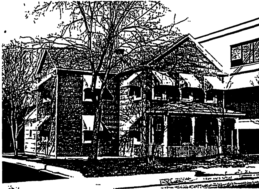
Figure 16. The Wells-Ulrich House: Lot 21, Palestine subdivision - 4906 Decatur Street (originally Wells Avenue) Cross-gabled frame dwelling built in 1903.
