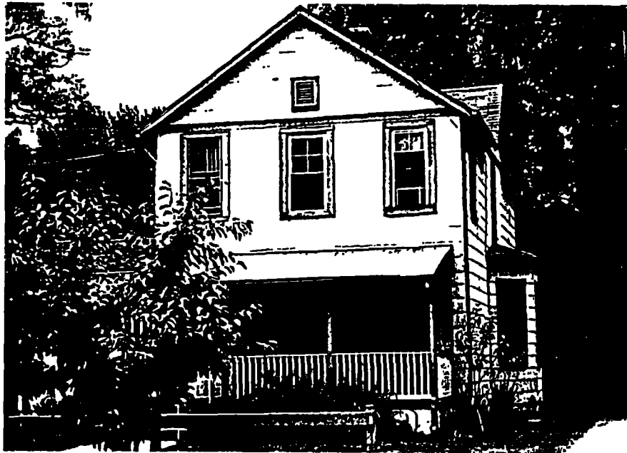
Figure 26. The Charles Norris House: Block E, Lots 2 and 3, Rogers subdivision 5103 Decatur Street (originally Wells Avenue) - Front-gabled frame dwelling built circa 1904 by Charles Norris.
