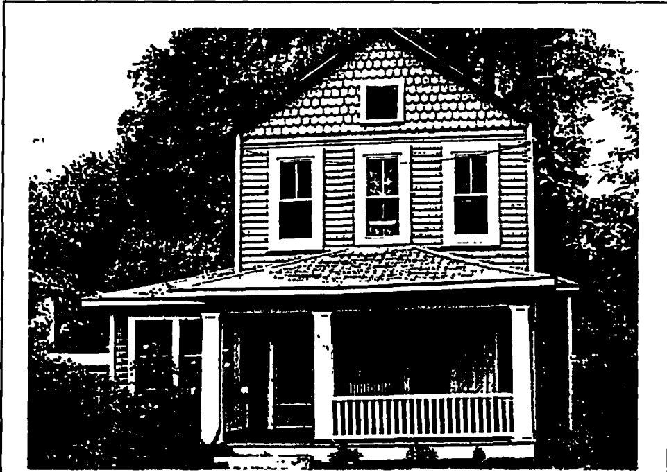
Figure 20. The Taylor-Blase House: Block E, Lot 4, Rogers subdivision - 5105 Decatur Street (originally Wells Avenue) Front-gabled frame dwelling built in 1900 by Elisha P Taylor.
