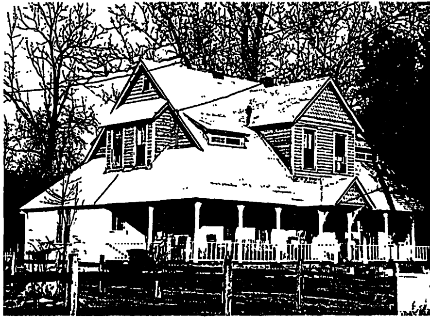
Figure 9. The Poppleton-Roberts House: 5104 Emerson (originally Washington) Street - unique house form in updated French Colonial style, built in 1901.
