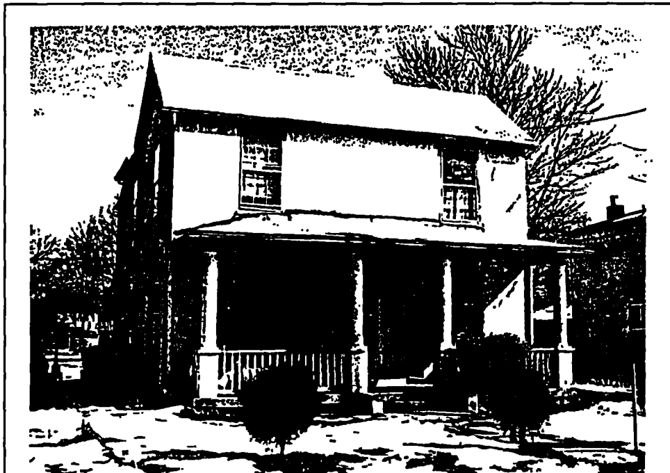
Figure 11. The Wells (rental) House: Lot 11, Palestine subdivision - 4905 47th Avenue (originally Charles Street) I-house type frame dwelling built by Dr. C.A. Wells in 1903.
